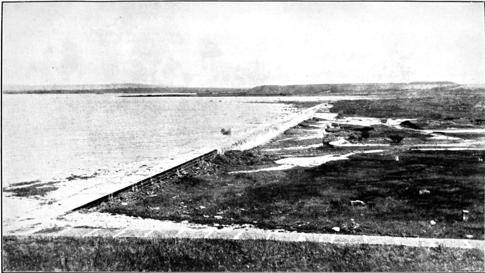
VISAPUR TANK. Waste Weir overflowing.
