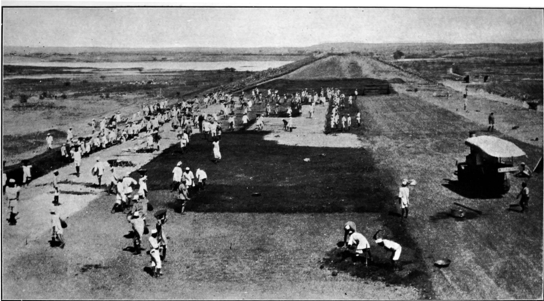
VISAPUR TANK. Convicts at work on the Dam.
