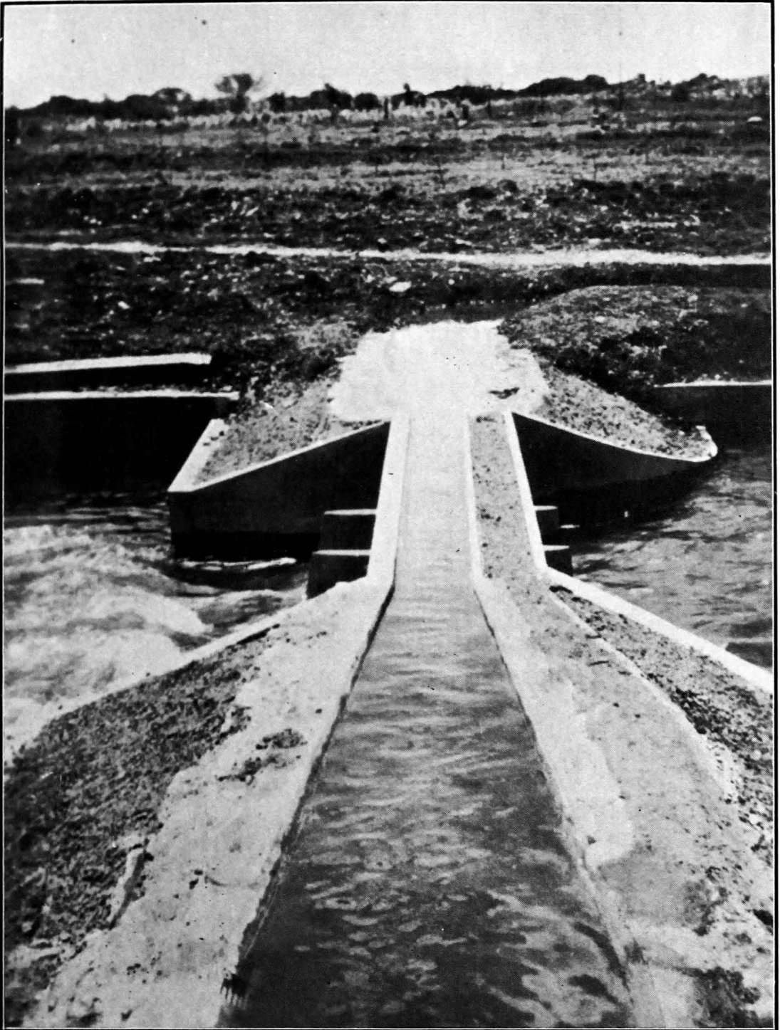
Model of Flumed Aqueduct No. 23. Bed width = 14 ft. Afflux = 0.166 ft. Full Size Discharge 474 Cusecs.
