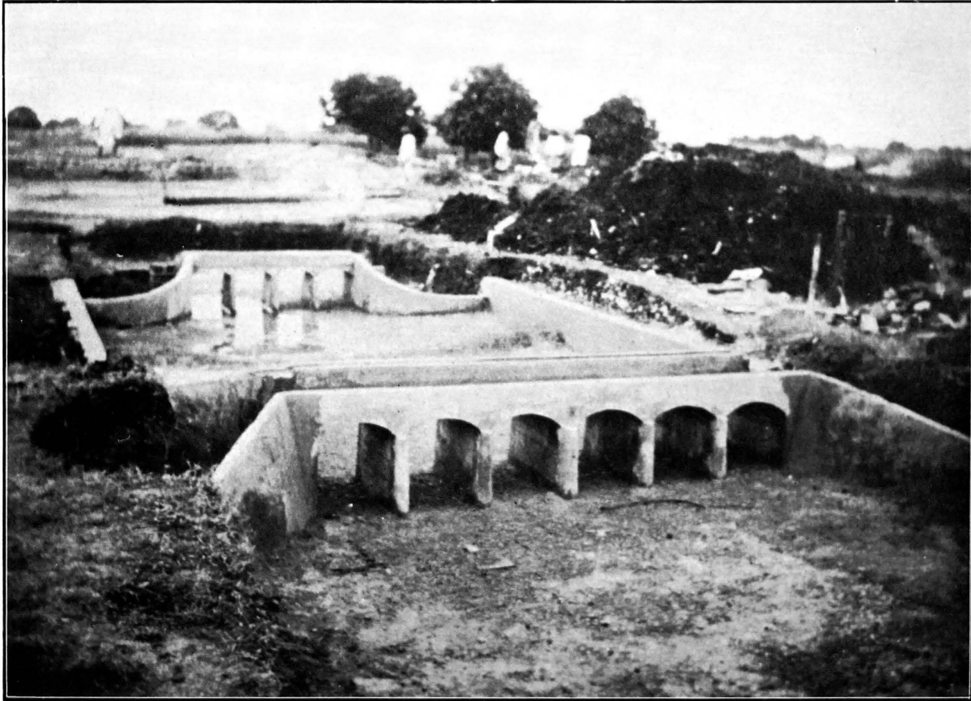
Models of aqueduct No. 23. Nira Right Bank Canal. (Under construction) Model Scale \frac{1}{24} .
