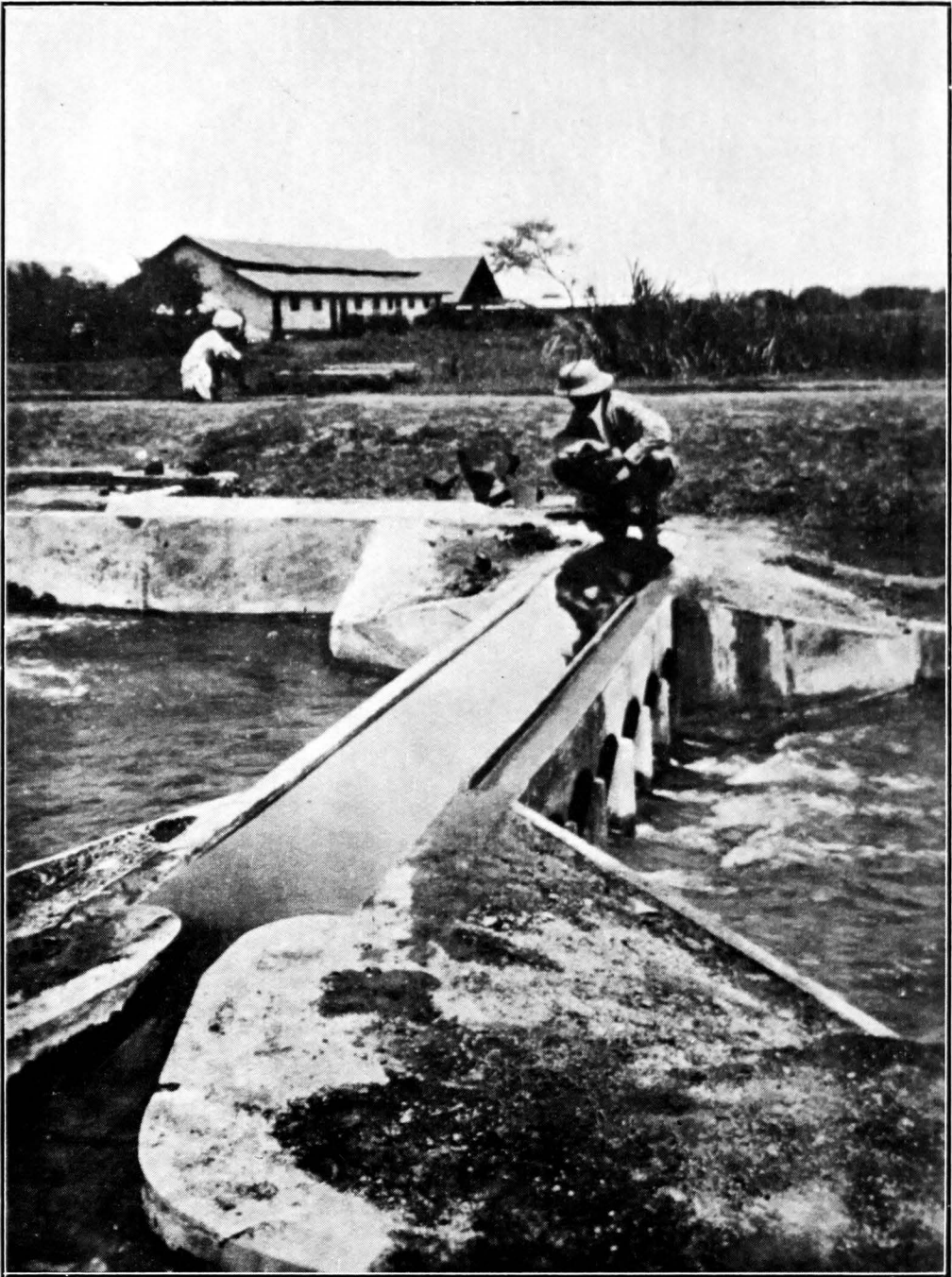
Model of Aqueduct No. 23. Nira Right Bank Canal as originally designed. Bed width = 34'—9". Full Size Discharge 474 Cusecs.
