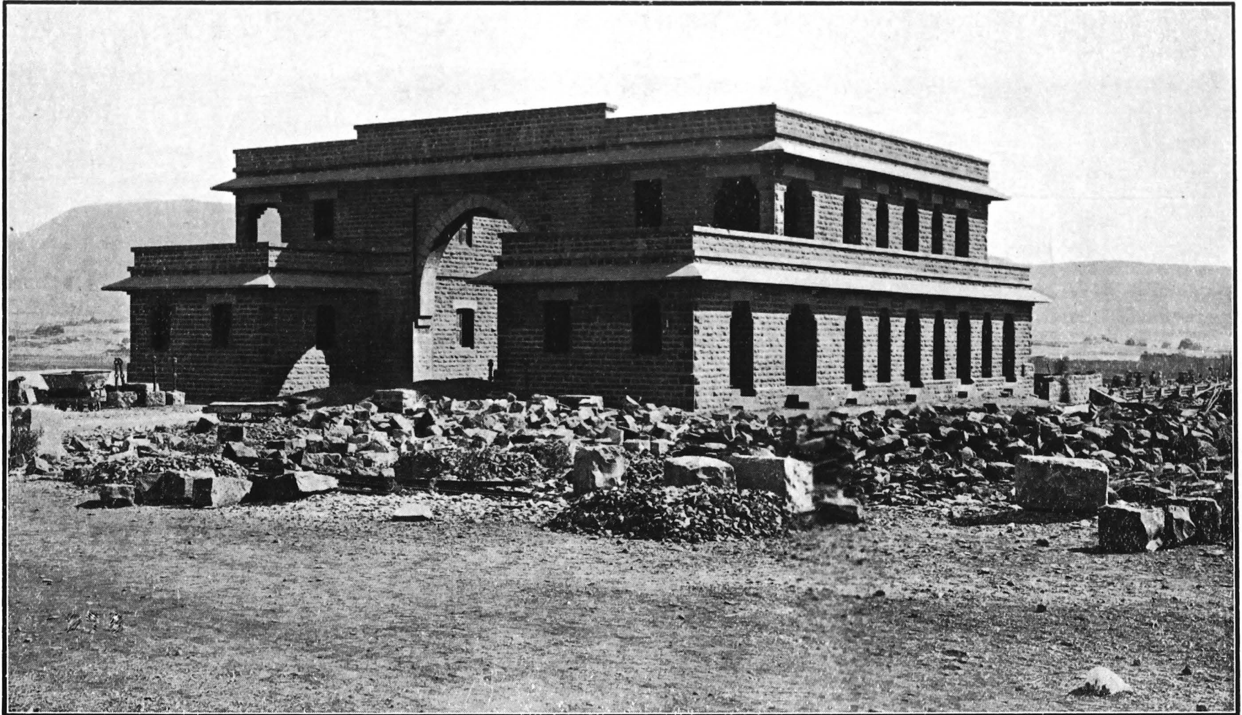
The Lloyd dam. Signaller's and Chowkidar's quarters at south end of dam. April 1925.
