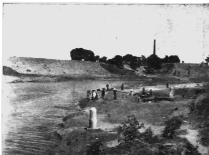
Photo No. 4025 : Kshipra at Ujjain. Photo looking upstream, showing the spur on right bank and fine silt deposit being removed from over the infiltration gallery. The concrete pillar seen in the foreground is constructed to locate the position of the gallery underneath.
