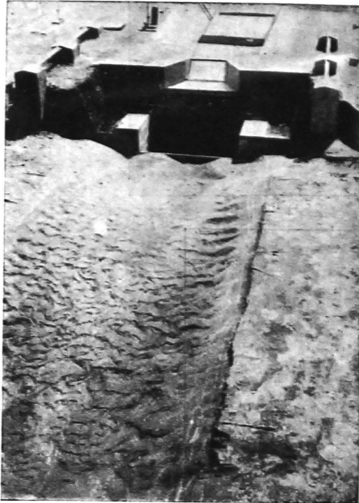
Photo 5142 : Photo showing final scour conditions when design in photo 5129 was tested with 25 per cent retrogression of downstream water-level. (The design consisted of a cistern \cong 21.34' wide; bed R. L. \cong 89.12 and deflector top at R. L. \cong 92. ).
