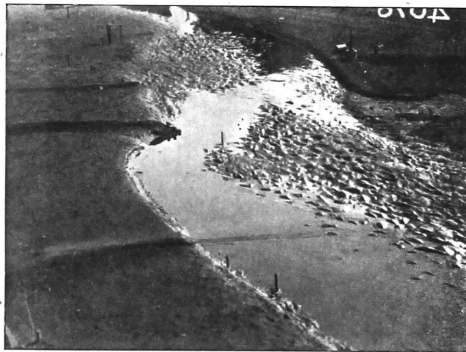
4076 Showing low water channel after experiment 12 with Barrage at Purana Killa and embankment as in experiment 11.
