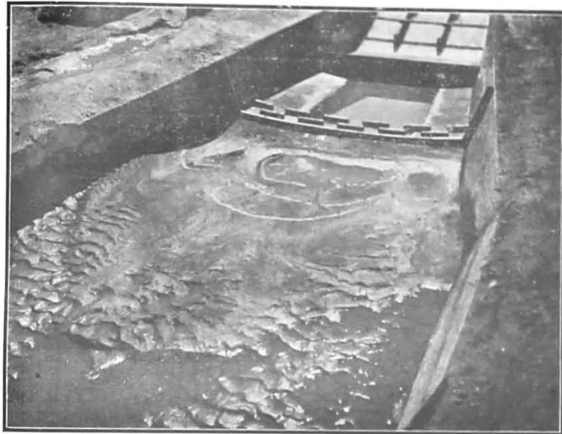
1848. Proportional Standing Wave Flume Meter Fall, Looking u/s, with baffle, deflectors and control blocks, showing scour d/s of the fall with 25 per cent. retrogression of d/s W. L. Looking upstream.
