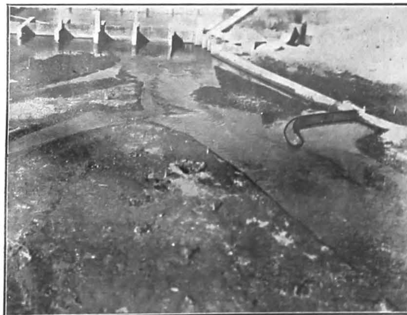
1891. Series VII, Experiment 3, with approved short spur at corner of the Right Afflux Bund, looking downstream.
