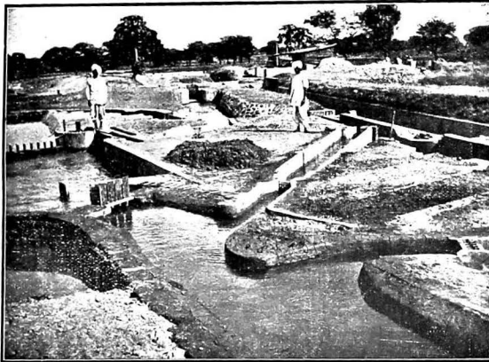
838. Experiment No. 2: (Looking downstream.) A spur projecting to midstream was built at the downstream end of the Mithrao to create curved flow to exclude bed silt.
