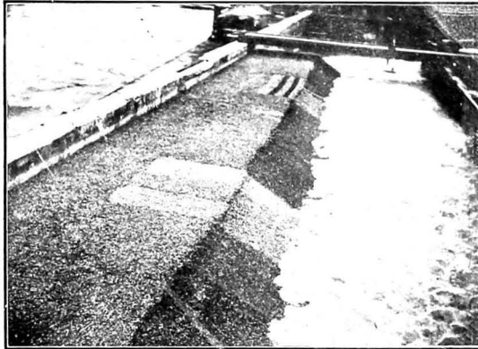
1167. Showing a falling apron experiment using different coloured pebbles to trace how "launching" takes place.
