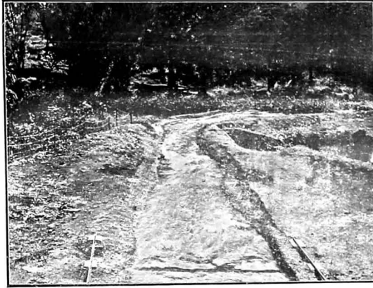
1575. Condition of flow in the waste weir tail channel—as designed, looking downstream, with Q \cong 12,500 cusecs.
