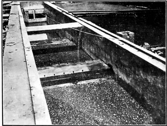
1390. Present design with faces of slabs at right angles to flow. Looking upstream.
