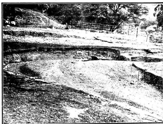
1539. Experiment 17 (1936 conditions). Looking downstream. Showing heavy scour of left bank upstream of ferry after 3 flood seasons.
