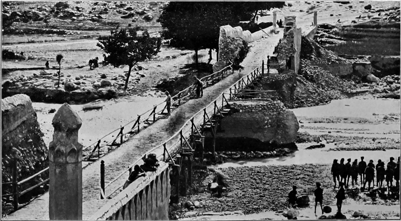
RESTORED BRIDGE OVER HASHIM KHEL STREAM, NEAR SAFED SANG (LOOKING EAST)
