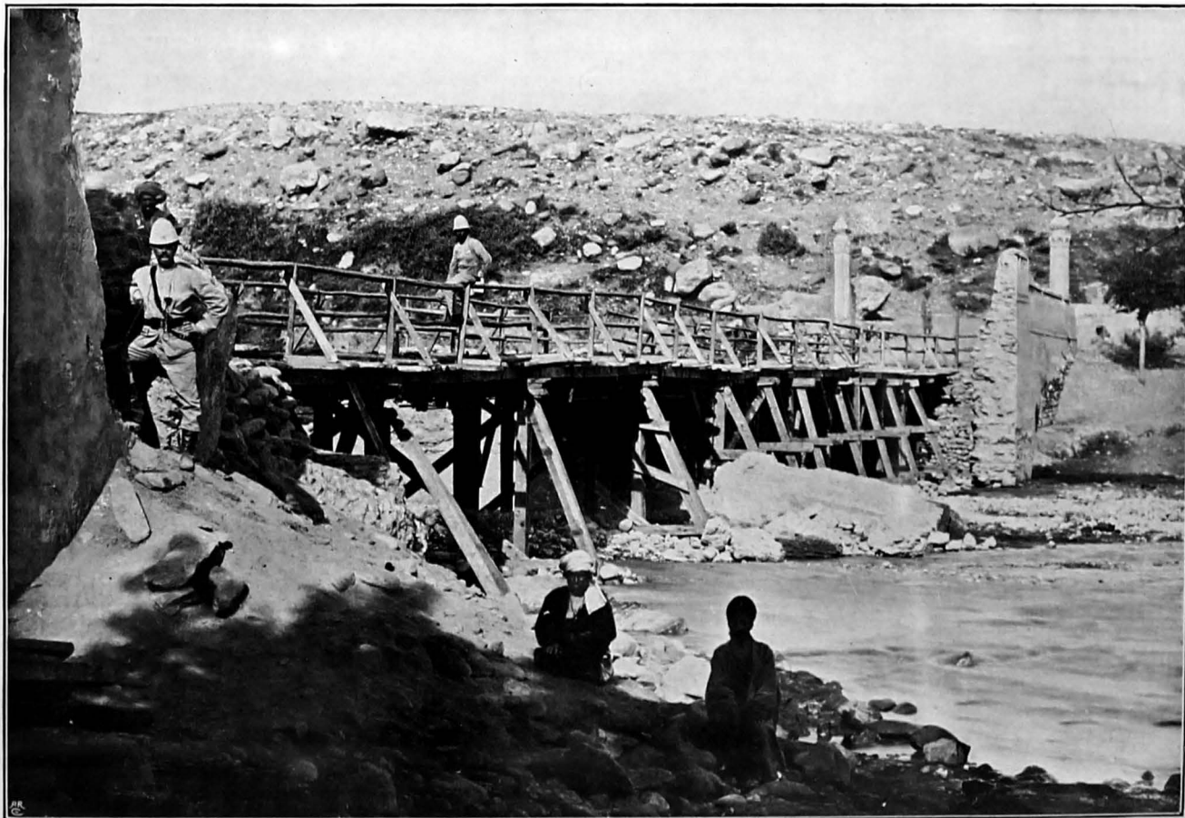
RESTORED BRIDGE OVER HASHIM KHEL STREAM, NEAR SAFED SANG (LOOKING WEST)
