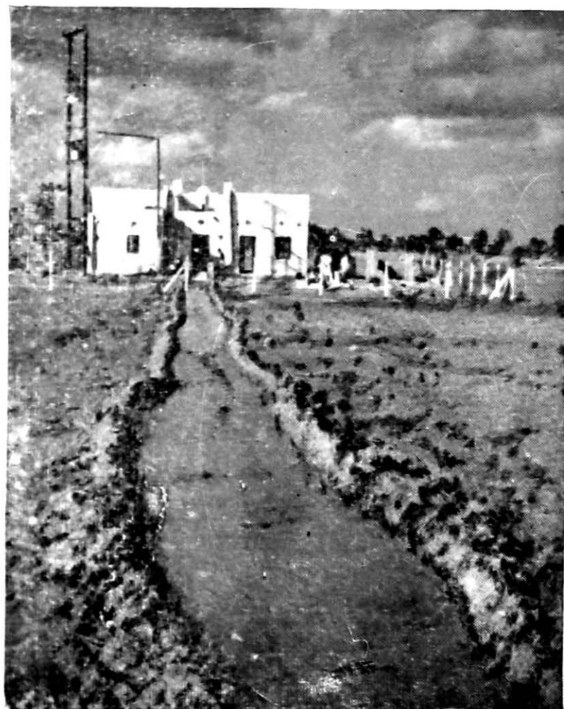
One of the Tube-wells in operation in West Bengal.
