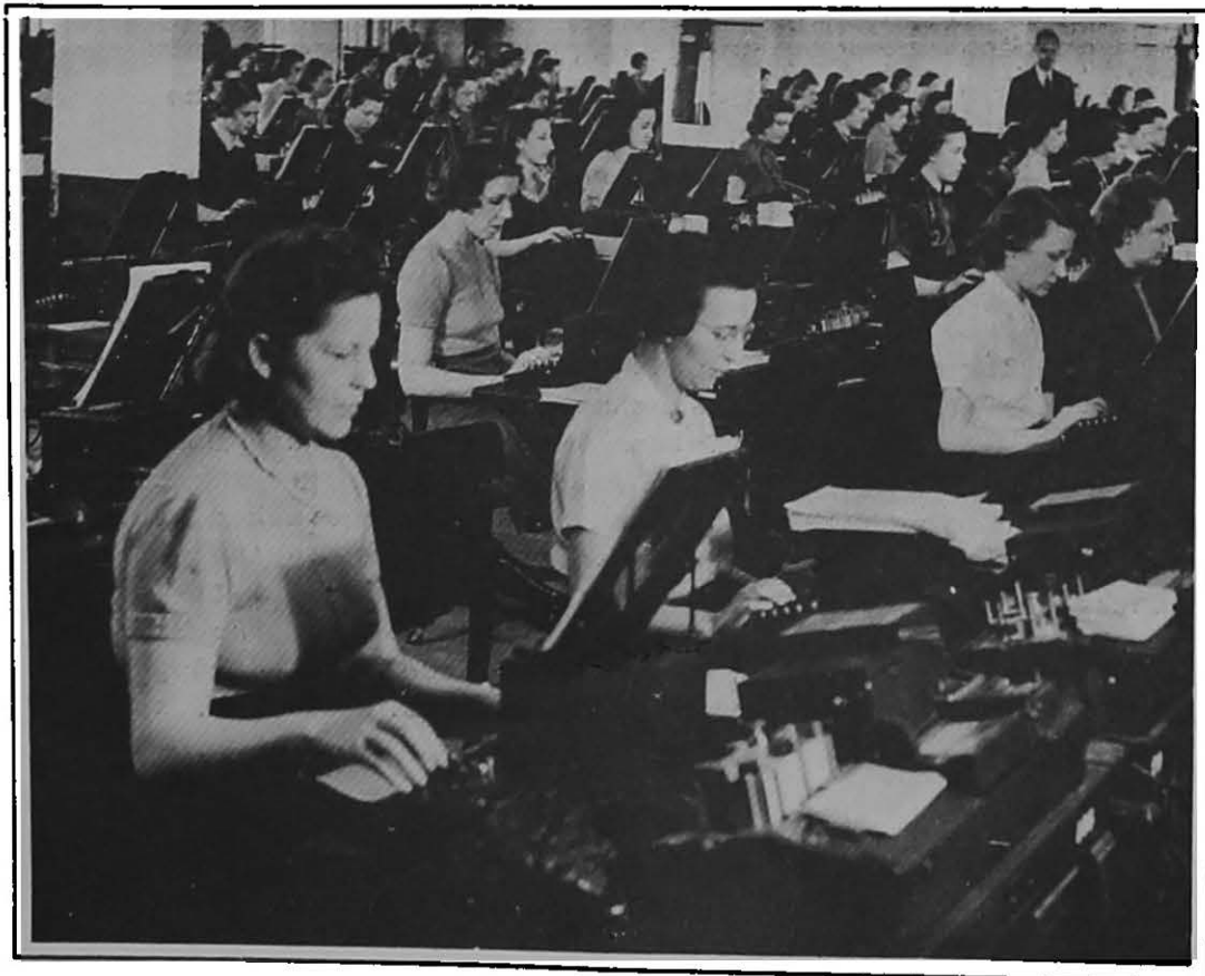
ONE SECTION OF THE CENTRAL PUNCHING UNIT
