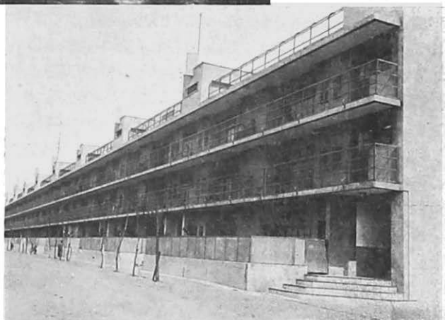
Married Workers' Apartment-House, Yodogawa
