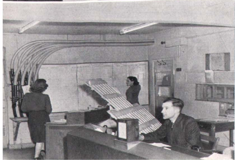
Keeping the Aircraft Movement Panel up to date in the Approach Control Room. The pneumatic tubes bring in messages from other rooms.
