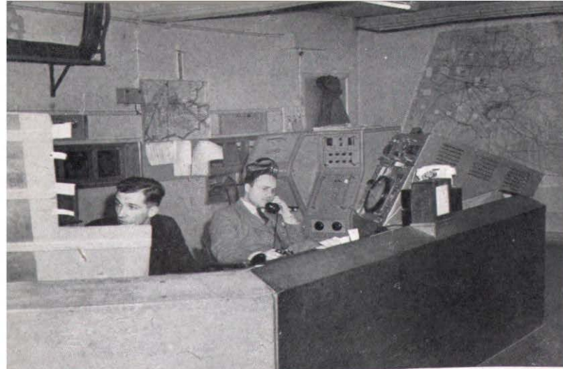
The Approach Controller's desk in the Control Tower. In the inclined case is the Airfield Control Radar tube.
