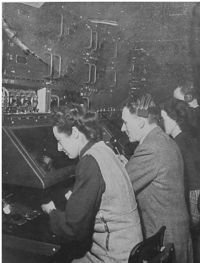
A part of the equipment used to help pilots to land. This is the Localizer Truck of the Instrument Landing System.
