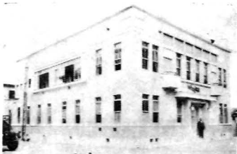
New Offices Recently Completed.
