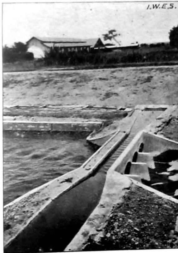
Photo 149. Aqueduct 23 as constructed. Width 14 feet.
