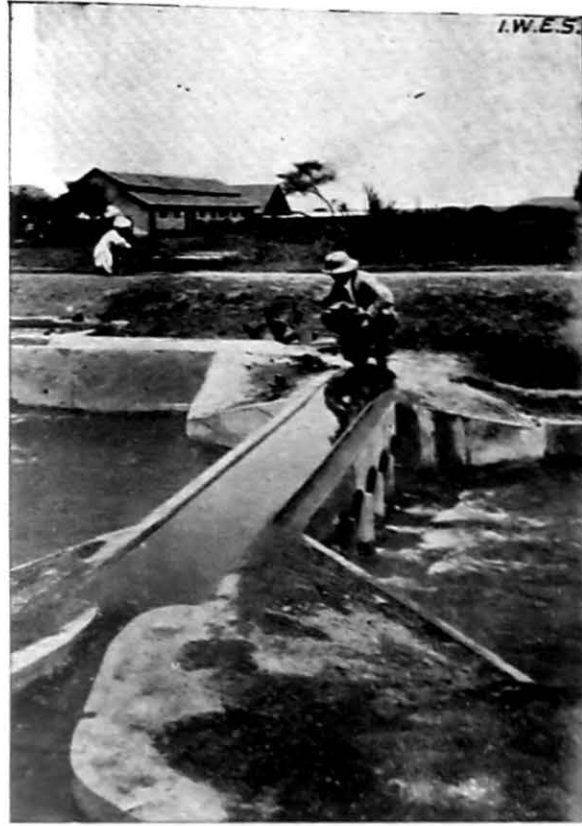
Photo 147. Model of Aqueduct 23, Nira Right Bank Canal, as designed. Full Supply Discharge \approx 474 cusecs. Width 34 feet.
