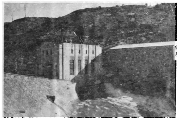
GRAND VALLEY POWER PLANT
