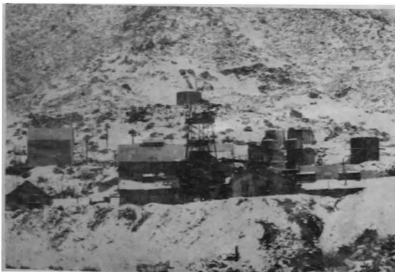
LEAD-SILVER MINE Power is supplied from Boulder and Parker Dam power plants on Colorado River
