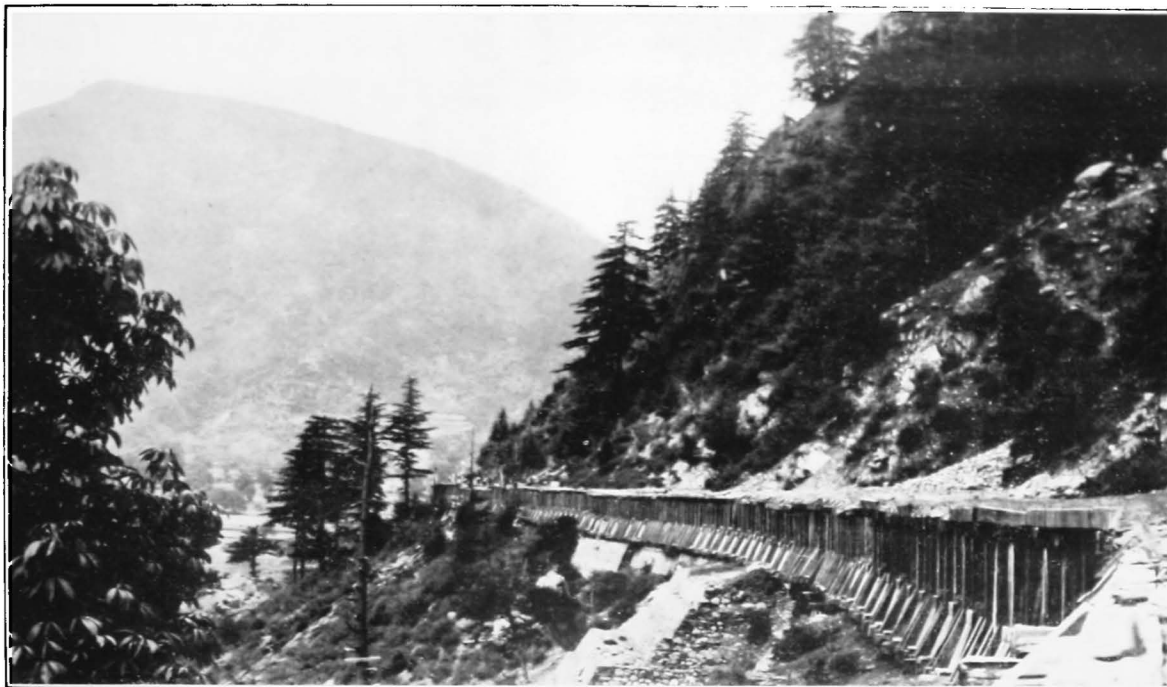
FLUME AT CHANANWARI, MOHORA. KASHMIR. JHELUM HYDRO-ELECTRIC INSTALLATION.
