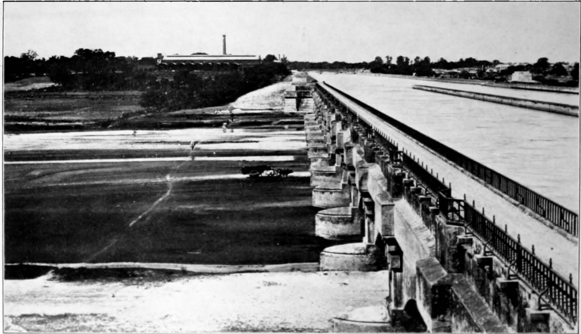
SOLANI AQUEDUCT, GANGES CANAL.
