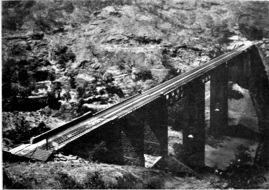
VIADUCT NEAR IGATPURI IN THE THAL GHAT, G.I.P. RAILWAY. Three 140-foot girder spans and four 40-foot arches.
