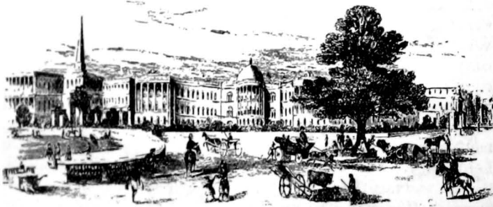
GOVERNMENT HOUSE AND TREASURY, CALCUTTA, FROM THE OLD COURSE. DESIGNED BY CAPTAIN CHARLES WYATT, B.E.
