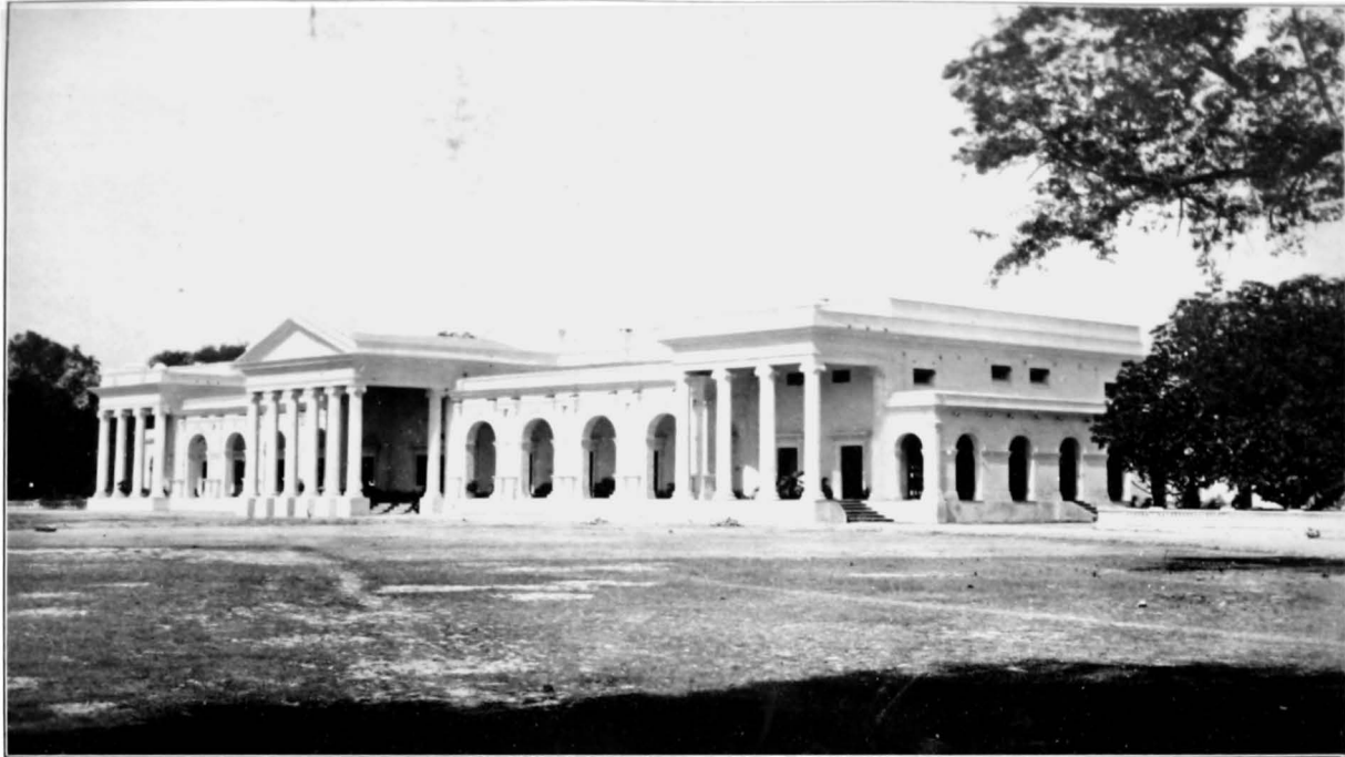
C.M.A.'S OFFICE, MEERUT, 1925-6, OLD BENGAL ARTILLERY MESS REBUILT. Originally designed by Captain G. F. Atkinson, Bengal Engineers (the author of Curry and Rice ).
