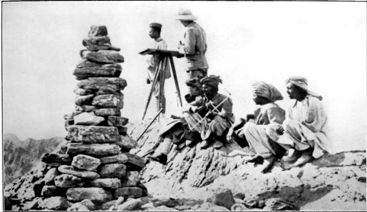
CHECKING A PLANETABLE.
