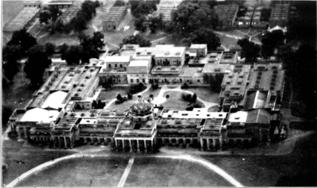
THOMASON CIVIL ENGINEERING COLLEGE, ROORKEE.
