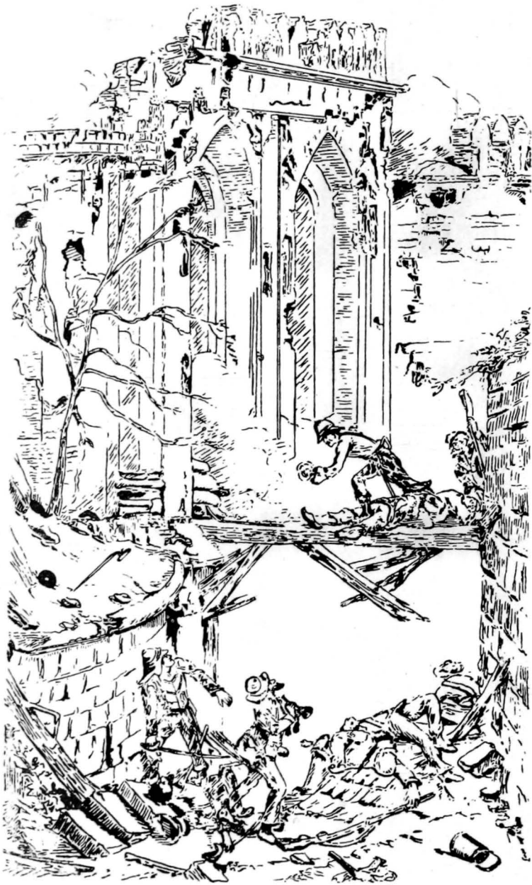
THE BLOWING IN OF THE KASHMIR GATE, DELHI, 14TH SEPTEMBER, 1857.
