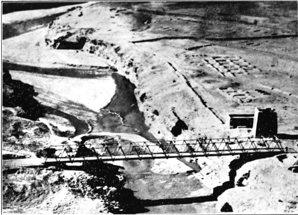
THE BARA BRIDGE ACROSS THE BARA RIVER, KAJURI PLAIN.
