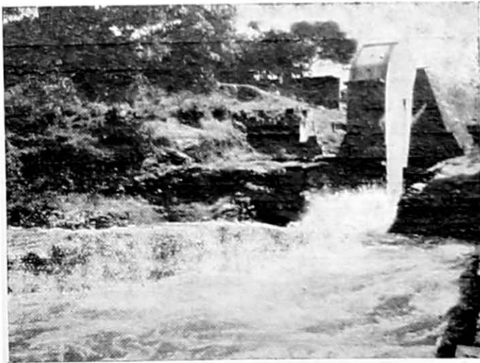
Model of 520-cusec Siphon Spillway
