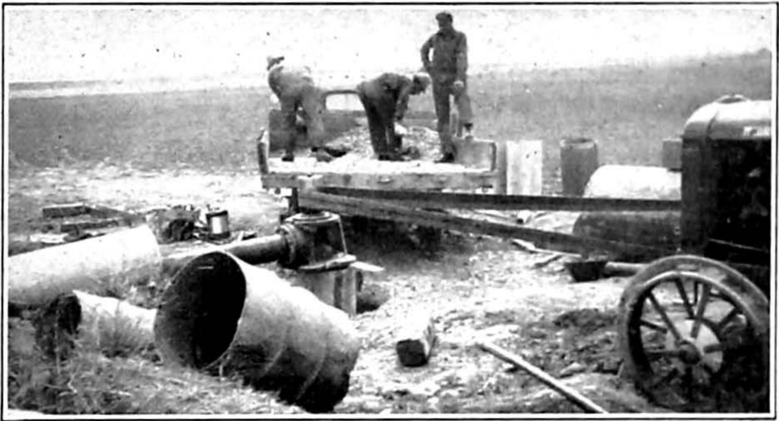
Figure 1.—Final stages of construction of an irrigation well. Applying gravel to outside of casing after removing larger outside blank casing and during test of well for capacity.
