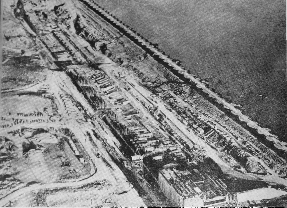
Fig 30 — The Longest Cofferd Dam with the Canadian-American Power House Link
