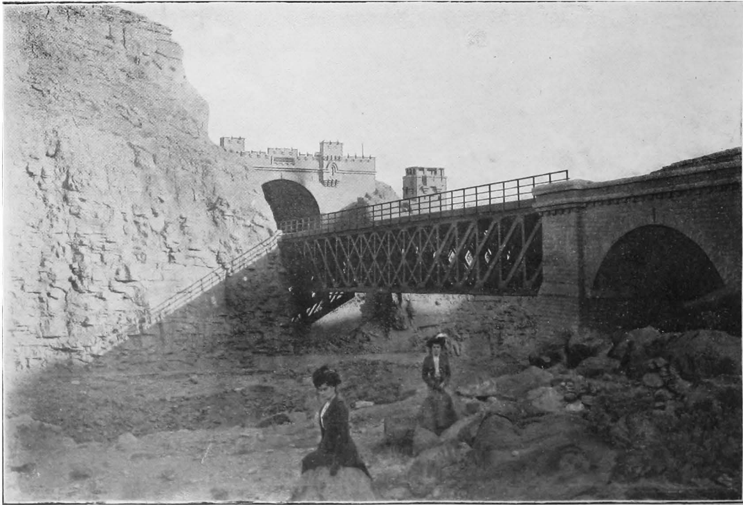
Mushkaf Bolan Railway. Pir Panja bridge.
