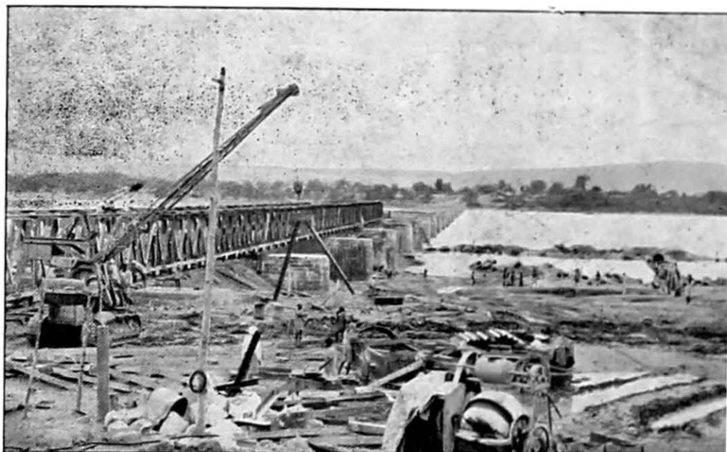
A view of the Rail-Road Bridge across the Mahanadi with Callendar Hamilton Bridge rolled in for a few spans. This bridge has since been completed.
