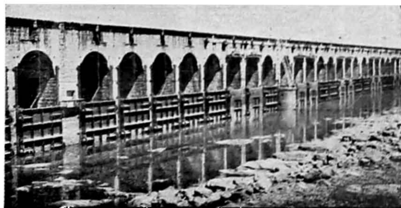
Automatic Gates Designed by Sir M. Visweswariah for the Khadakvasla Dam
