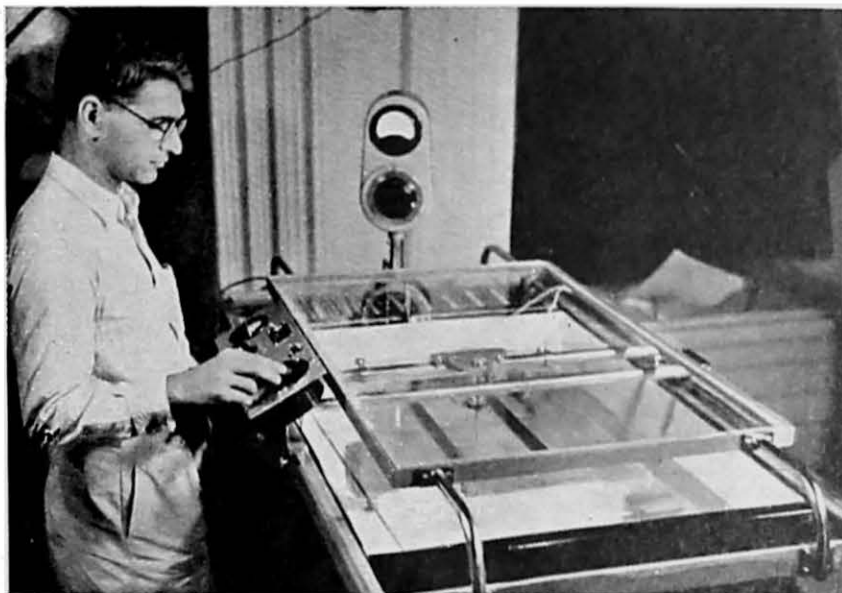
Apparatus for Determining Stress Distribution in Structures
