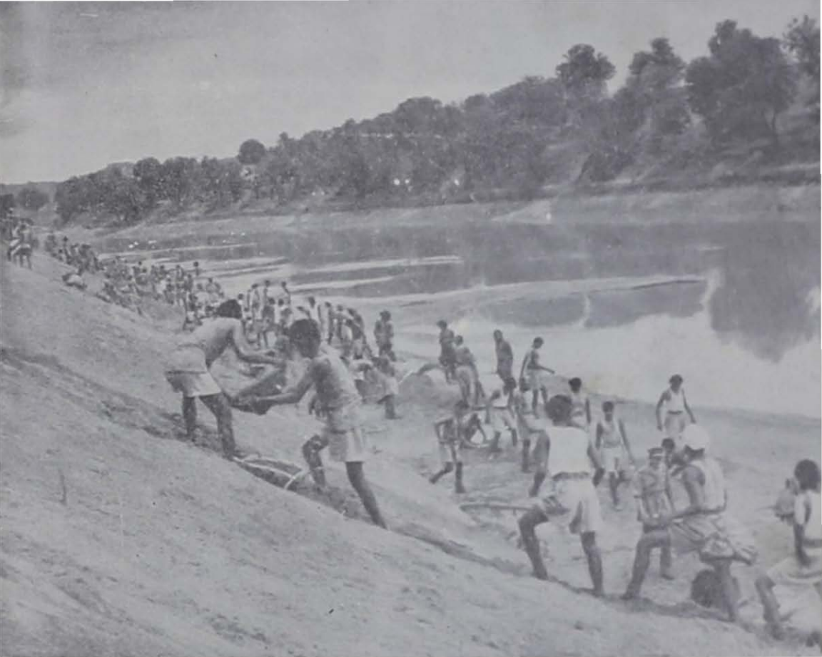
Widening the Sirhind canal for irrigation
