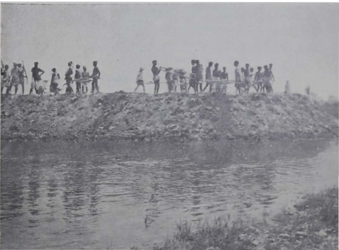
A bund being built round a tank
