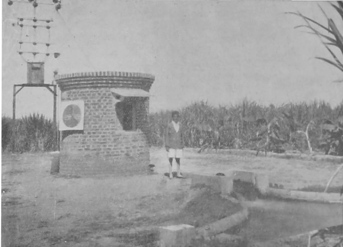
A tube-well with a measuring tank
