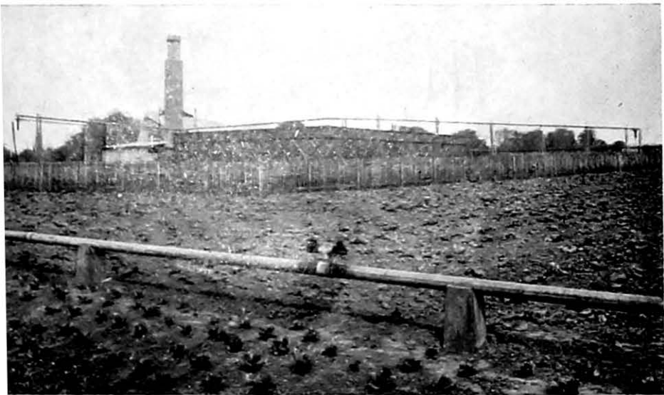
FIG. 9. General view of irrigation power plant, with storage tank.
