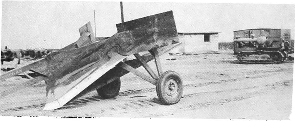
Photograph No. 57 Canal excavator used by a canal lining contractor at Phoenix, Arizona.
