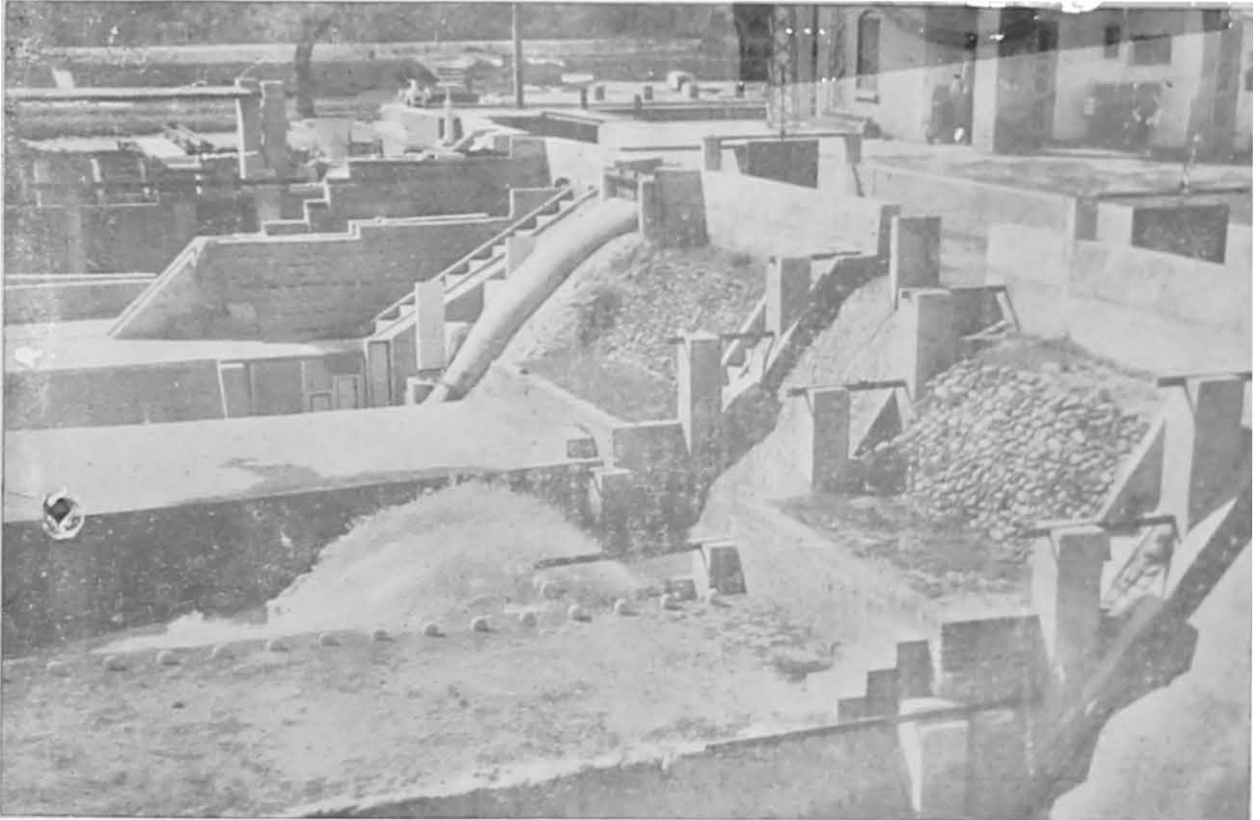
Model studies of the Spillway of the Bhakra Dam Shooting bucket in operation
