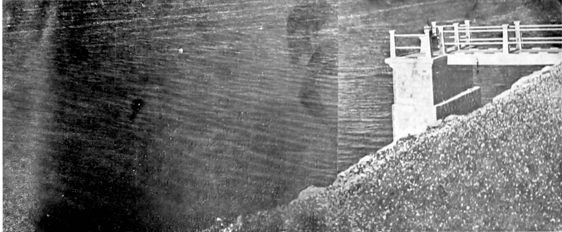
The Dukrikheda Tank (Hoshangabad)
