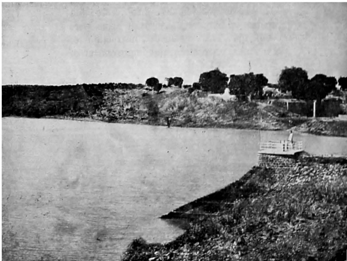
The Ramaua Tank (Gwalior)
