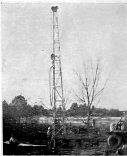
FIG. 7. Modern well-drilling rig drilling irrigation deep well. (Note rig is mounted on bed of truck.)
