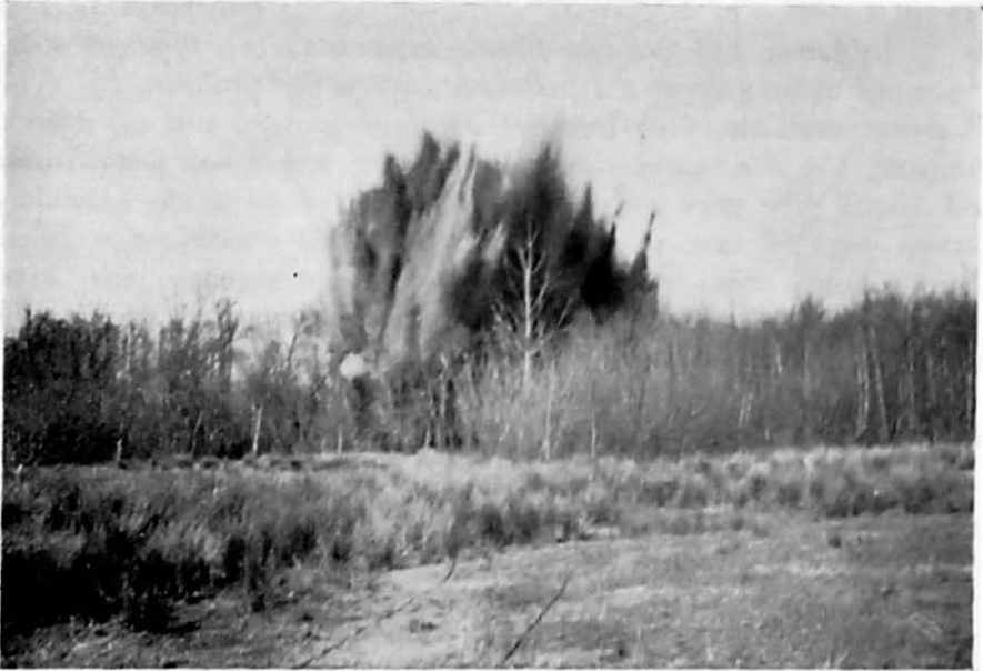
FIG. 17. Ditching dynamite can be used effectively in all sections of the State if blasting is done when soil is in saturated condition.
