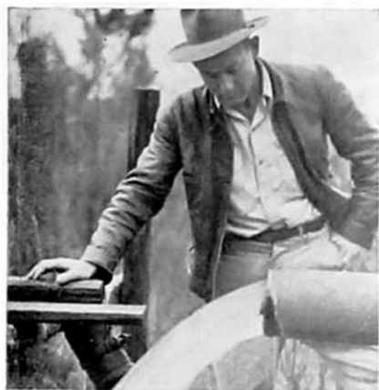
FIG. 5. Flowing artesian well discharging 225 gallons per minute (13,500 gallons per hour.)
