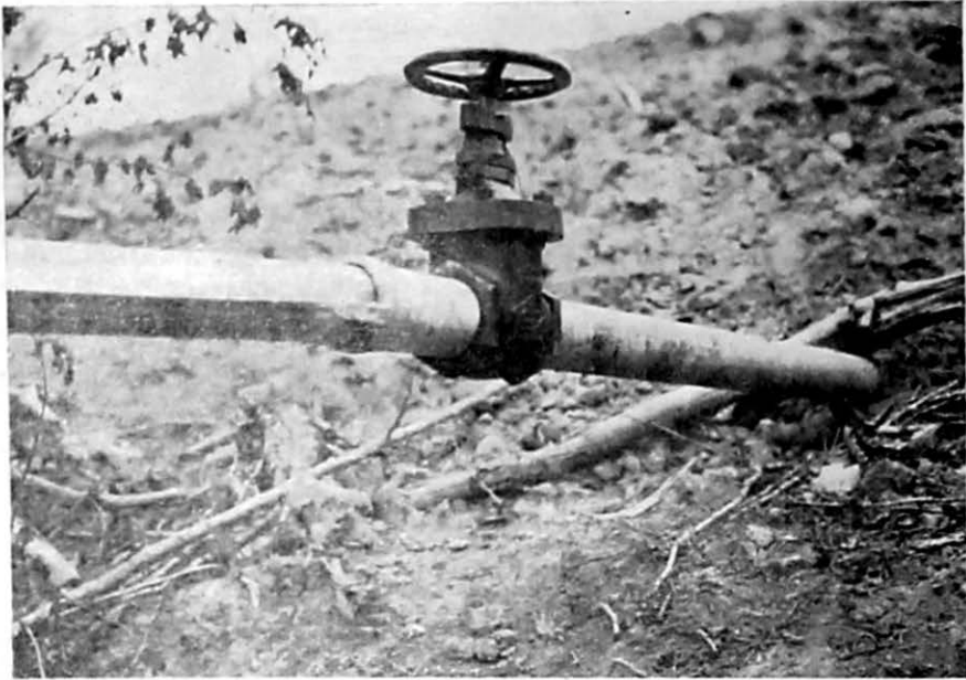
FIG. 4A. Irrigation pipe connected to drain pipe in dam with simple adaptor unit. Valve controls flow of water.
