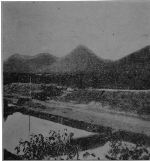
FIG. 32.—Borrow pits on the Raipur-Vizianagram Railway, freshly excavated. A. vagus only.
