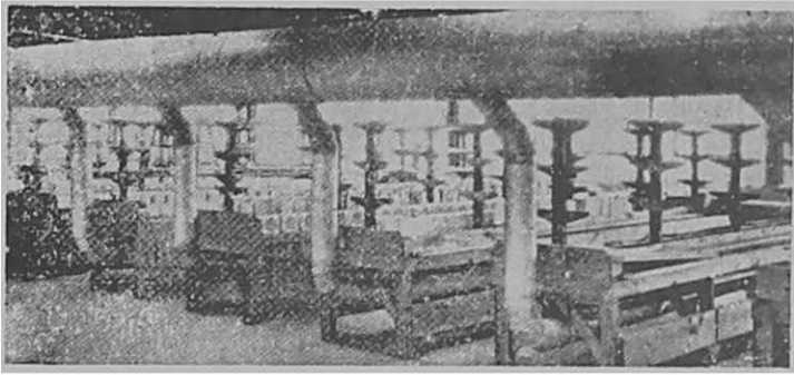
A Waste Heat Drier
