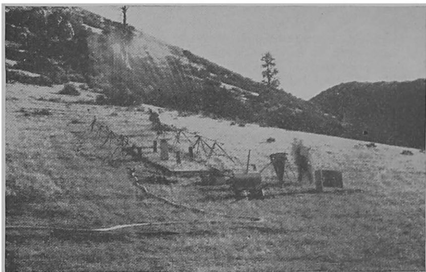
FIGURE 14.—By using a portable artificial "rainmaker" it is possible to obtain run-off data for rains of different amounts and intensities under a variety of conditions.
