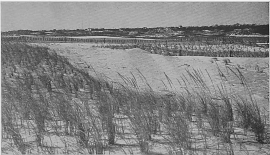
Figure 30. Picket fences and planted beach grass used to hold the sand in place. Note the drift held by the fence.
