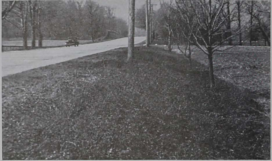
Figure 22. Highway shoulder protected by trailing honey suckle ( Lonicera japonica Halliana ).
