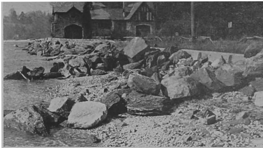
Figure 38. On the north shore of Long Island. Boulders being used as jetties to protect the road at right.
