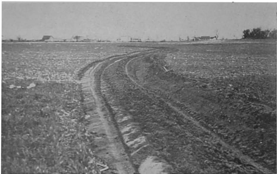
Figure 13. Terracing with a blade terracer. Here is shown the beginning of the operation of moving soil to form a terrace channel and embankment. Two cuts have been made with the blade.
