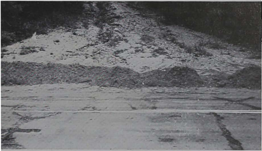
Figure 21. Sand and gravel washed down a side road. This too has been cleared off the concrete with a road grader.
