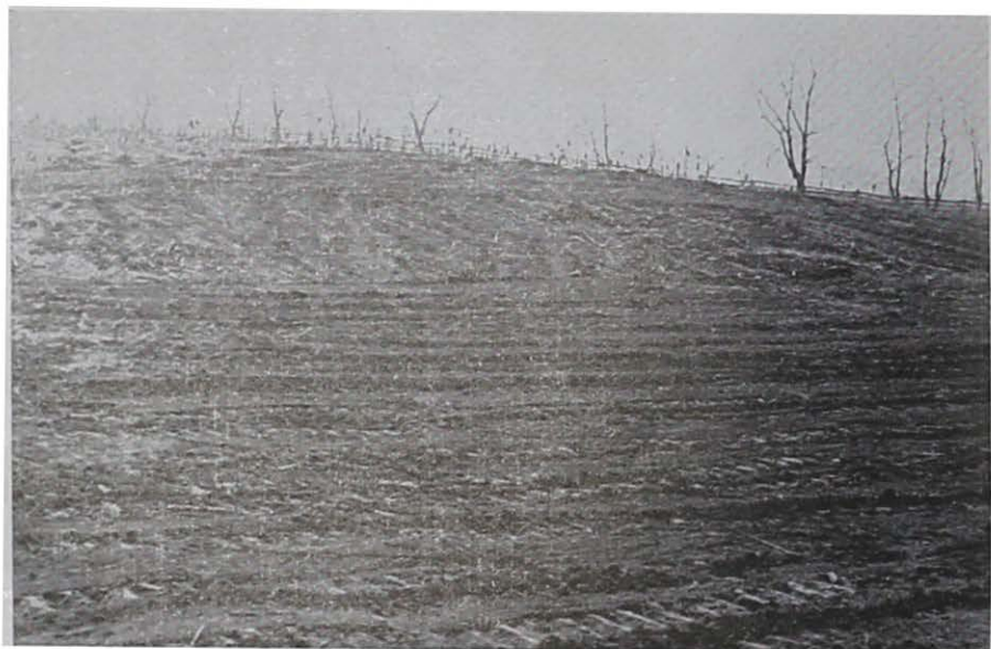
Figure 6. Filled gullies. Here a bulldozer has been used to push eroded soil back up onto the slope and to fill gullies. This practice is seldom followed in this country.
