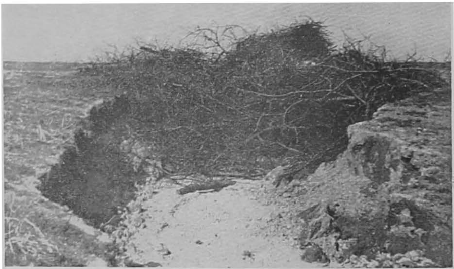
Figure 9. Brush piled in gullies to check their growth—too little too late.
