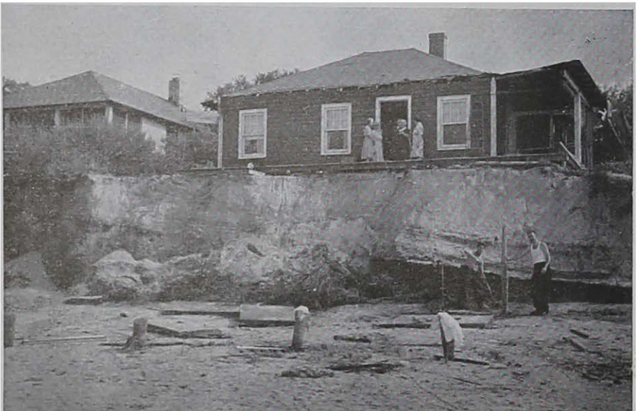
Figure 35. Same cottage as shown in figure 34. Photographed after the hurricane of September 14, 1944. About 40 feet of shoreline was cut away by the waves. Similar damage was done under like conditions in many places along the north shore of Long Island.
