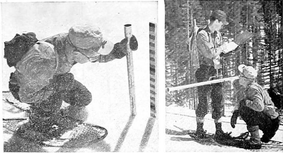
FIGURE 8.—The Utah snow sampler was used to take samples of snow depth and water content at 25 points on each plot.
