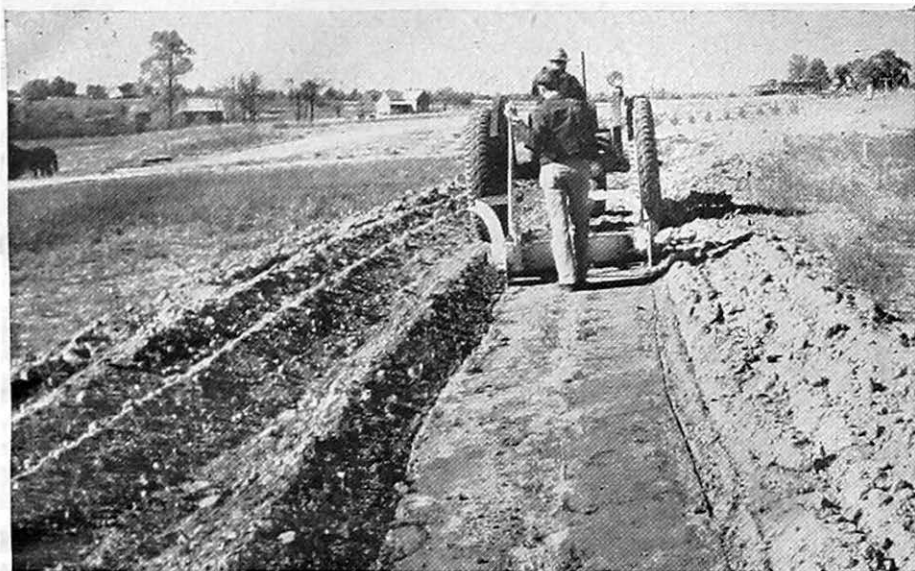
FIGURE 25.—Terracing with a light blade and farm tractor.
