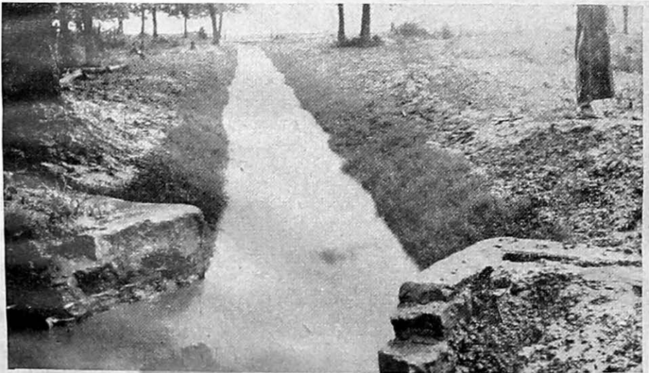
FIGURE 17.—Constructed terrace outlet stabilized with Bermuda grass. Velocity of the water is 7\frac{1}{2} cubic feet per second.
