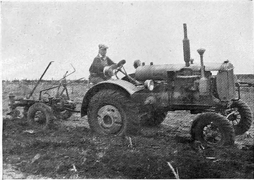
FIGURE 21.—The rotary-type terracer developed by the Agricultural Engineering Department of Iowa State College.
