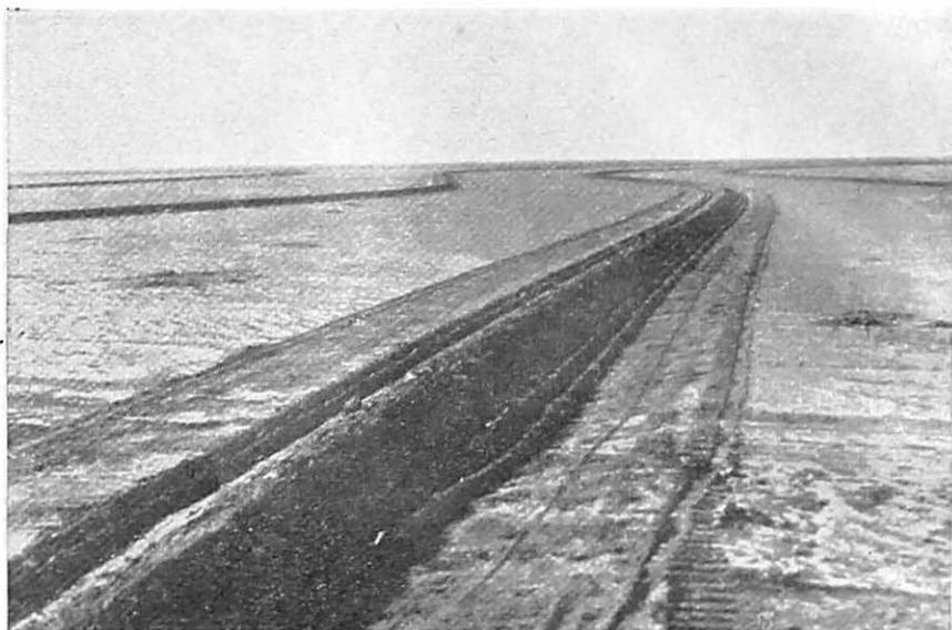
FIGURE 23.—Partly constructed ridge terraces in the Great Plains, where slopes are relatively flat and uniform.
