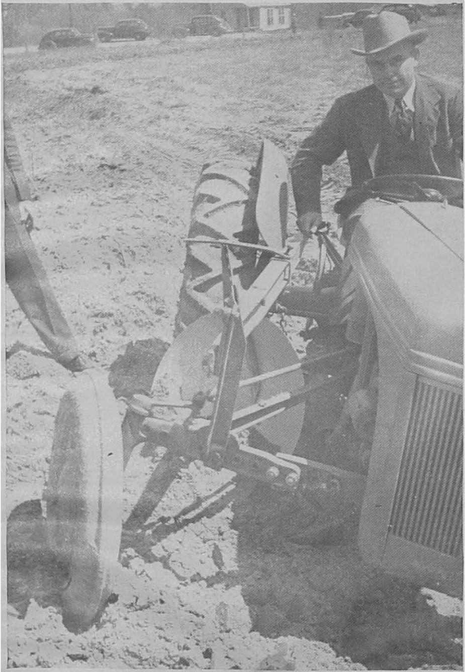
FIGURE 31.—A special disk attachment for farm tractors has proved efficient for terrace construction.
