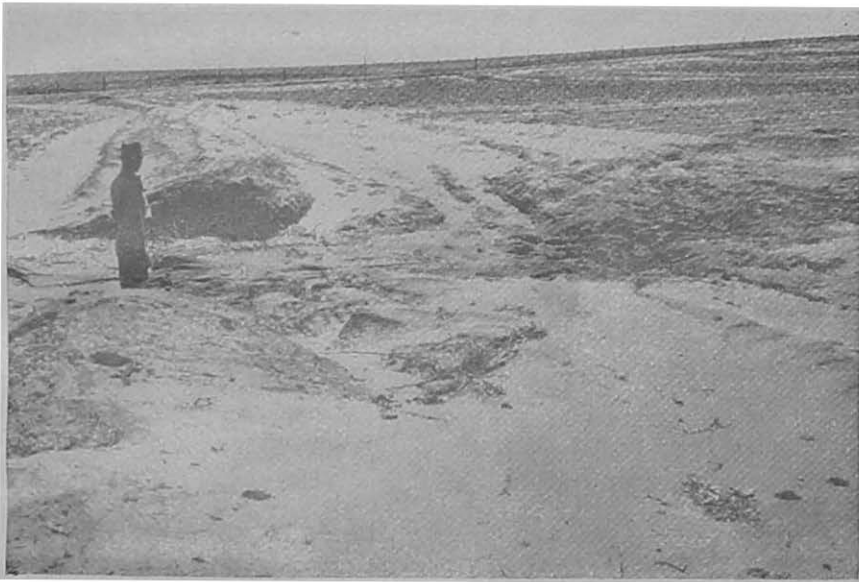
FIGURE 6.—Overtopping, caused by improper design, construction, or maintenance of terraces, damages both field and terrace.
