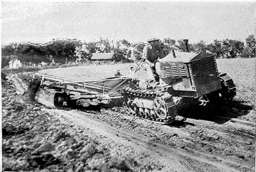
FIGURE 22.—The elevating-grader terracer developed by the Agricultural Engineering Department of the University of Missouri.
