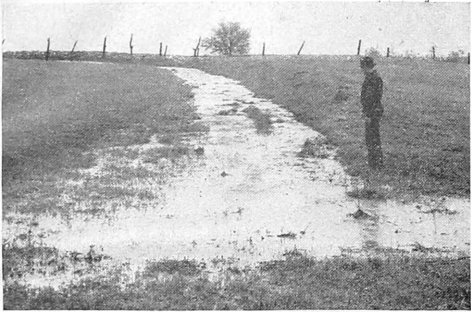
FIGURE 16.—A terrace discharging onto pasture sod. The water spreads as it leaves the terrace channel. Much of it will be absorbed and stored in the soil.
