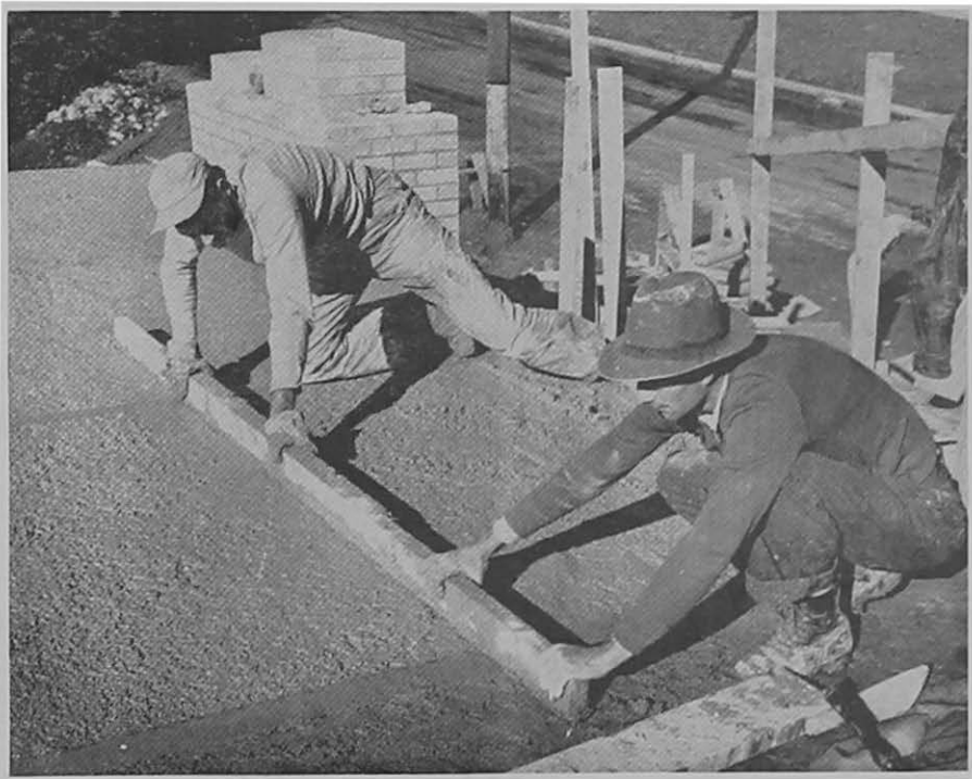
Figure 4.—Roof slab of wood-waste concrete. The screeding operation shown above was followed by smoothing with a steel trowel in 3 hours. Built-up roofing was then applied directly to slab.
