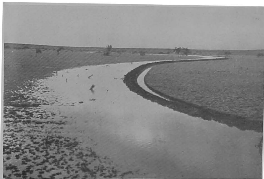
On range areas, structures are built to spread water over the land.
