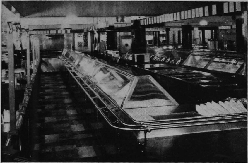
Courtesy Forum Cafeteria Systems
