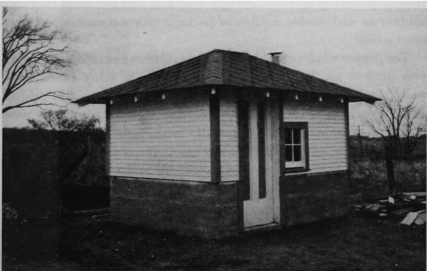
Figure 7. Milk house of frame construction. Note impervious foundation walls
