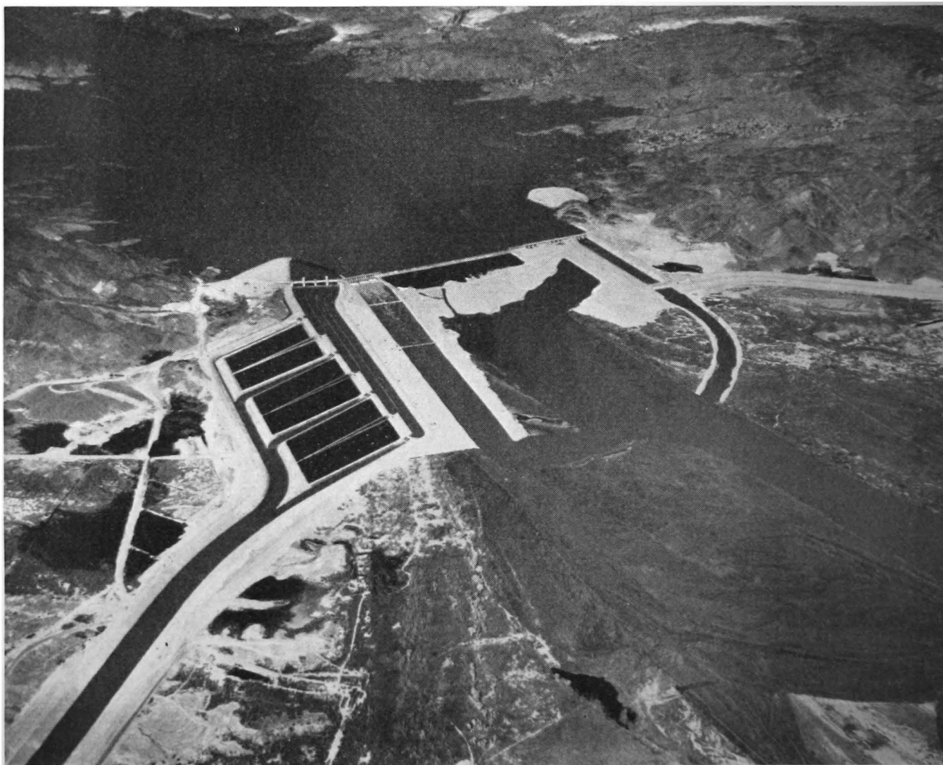
FIGURE 18.—Imperial Dam, Desilting Works, and All-American Canal
