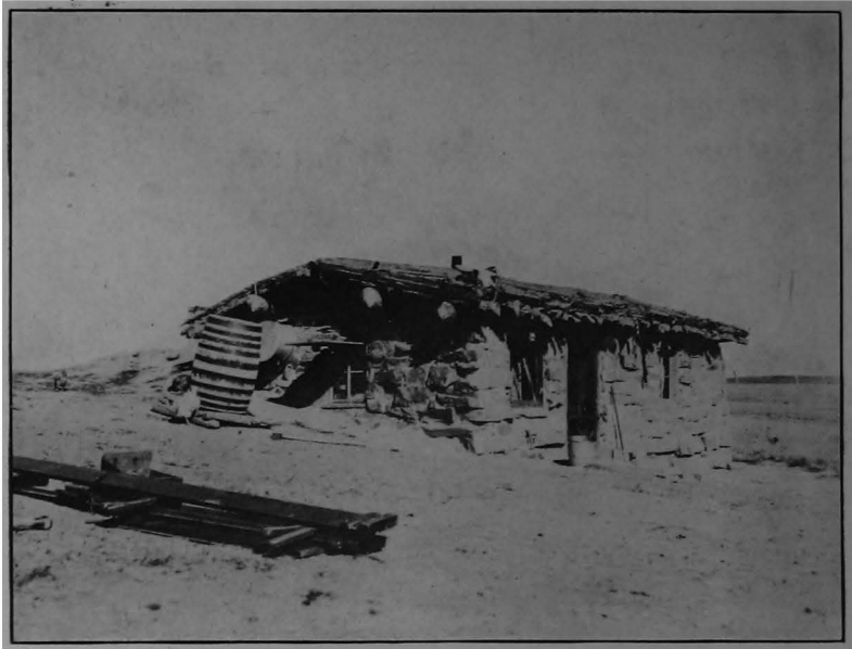
STONE HOUSE. NOTE BUFFALO SKULL ON ROOF.
