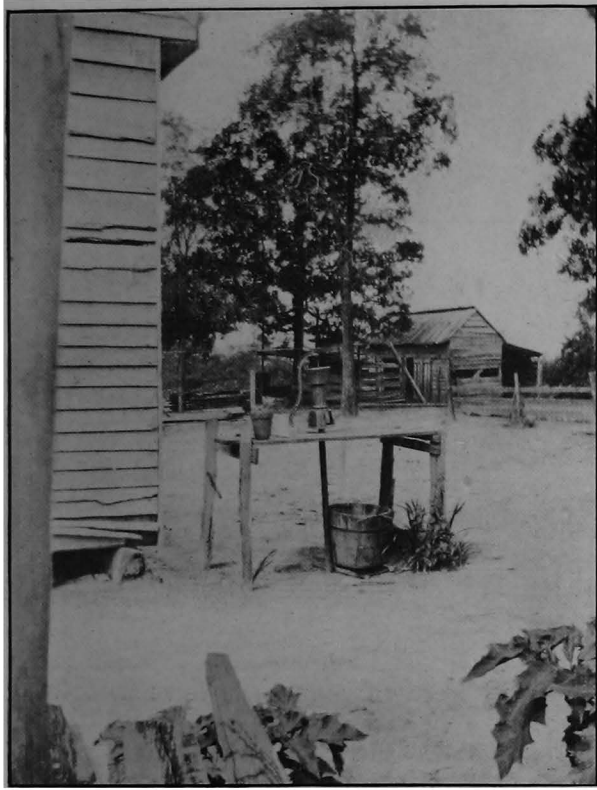
PLATE XII.—DRILLED WELL CONVENIENTLY NEAR THE HOUSE.
