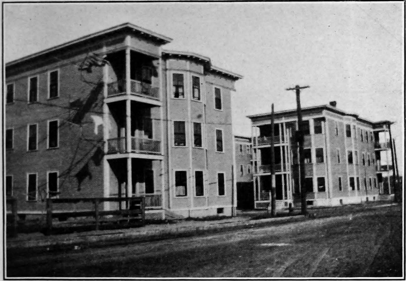
PLATE I.—TENEMENT HOUSES IN THE FOURTH WARD, OUT TOWARD VALLEY STREET. MODERN PLUMBING, TOILET ON EVERY FLOOR, ALL SIDES EXPOSED TO LIGHT AND AIR. TYPE OF TENEMENT HOUSE BECOMING MORE COMMON IN MANCHESTER.
