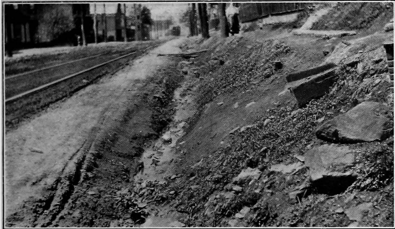
OPEN DITCH ALONG WOODVALE AVENUE, WHICH RECEIVES ALL KINDS OF HOUSE DRAINAGE.
