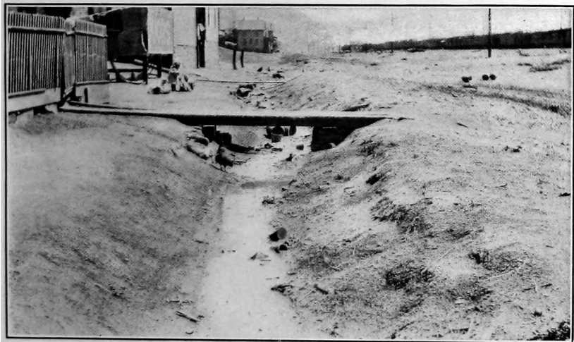
VIEW OF AN OPEN DITCH ON PLUM STREET, WHICH RECEIVES HOUSE DRAINAGE OF ALL KINDS.
