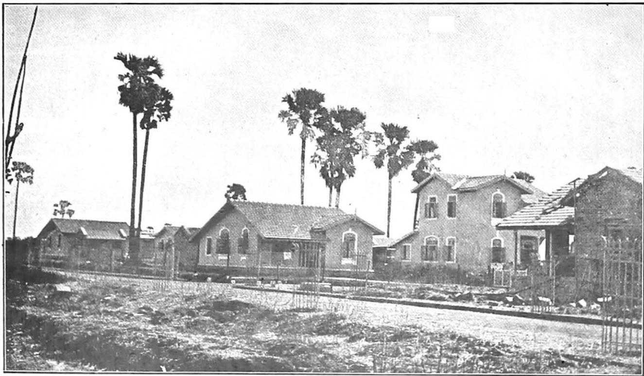
Typical cottages erected in S.S. No. 7, Khar.
