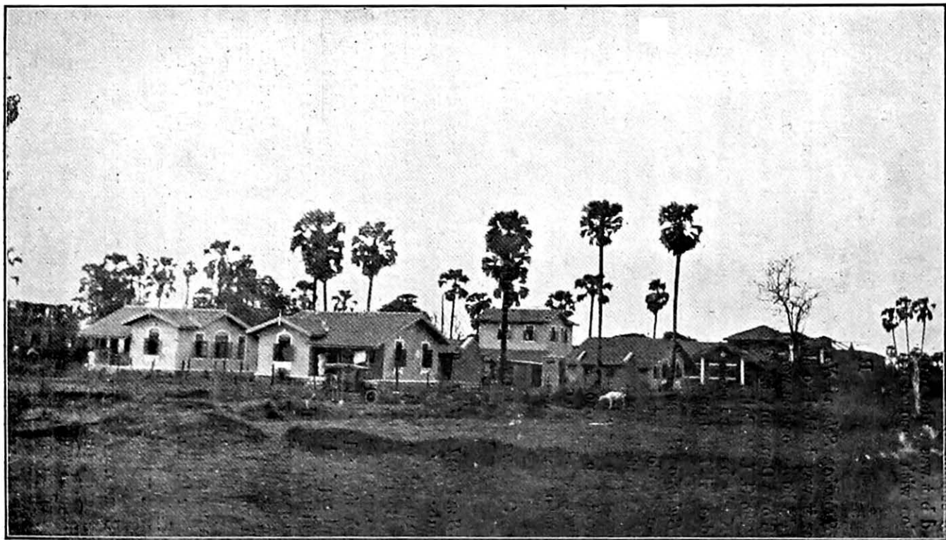
Typical cottages erected in S.S. No. 7, Khar.
