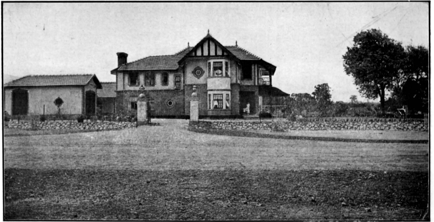
Suburban Scheme No. 3 (Chembur Section "A"). Bungalow (cost Rs. 42,000) erected in the Garden Suburb by the Development Directorate. Date 3rd April 1924.
