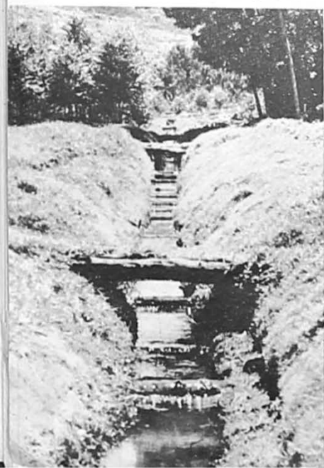
African swamp reclaimed by run off channels which are stepped to prevent gullying.
