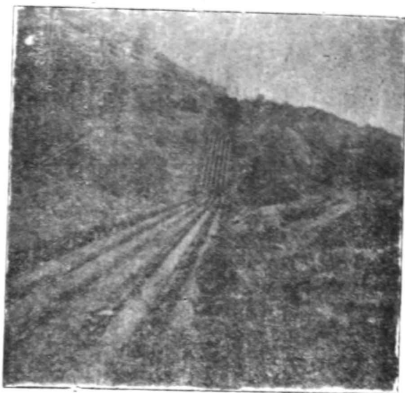
Pipe line of the Tata Hydro—Electric Scheme, Bombay.
