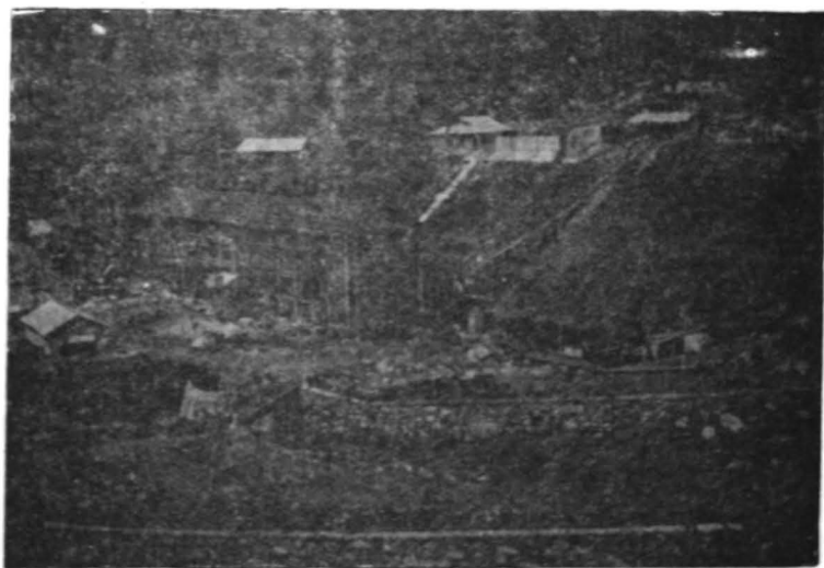
The Mandi Hydro-electric scheme—Power House at Jogindernagar.
