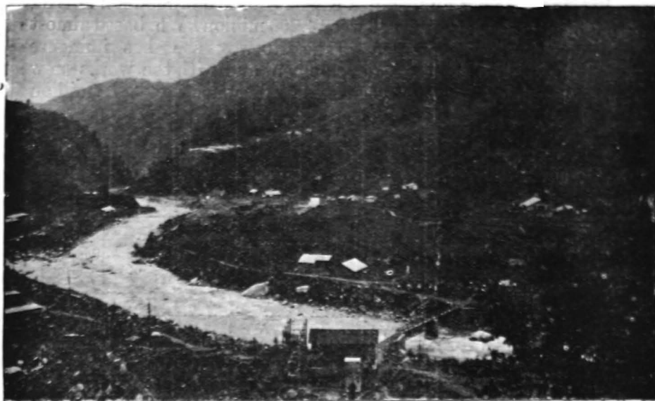
Mandi Hydro-electric Scheme—Head-works area looking South.
