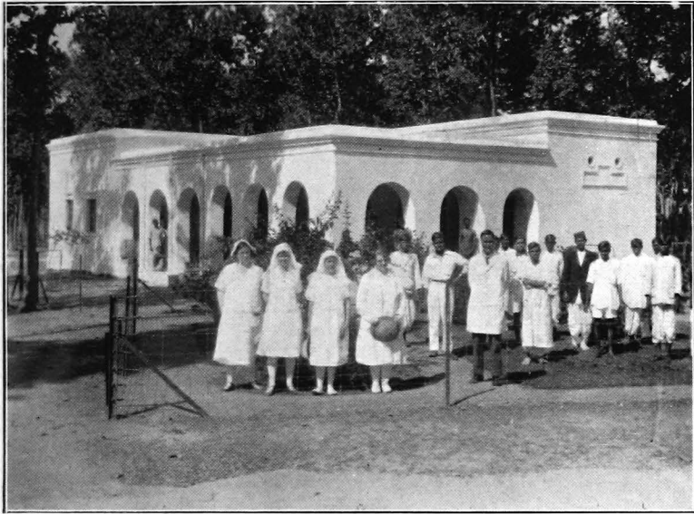
The recently completed Treatment and Research Block at the Purulia Leper Colony. Members of the healthy and leper staff are shown in the foreground and also two ladies training for work in South India.
