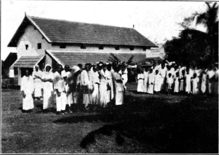
Among the new buildings erected during the year are these additional quarters for women patients at the Calicut Home, Madras Presidency.
