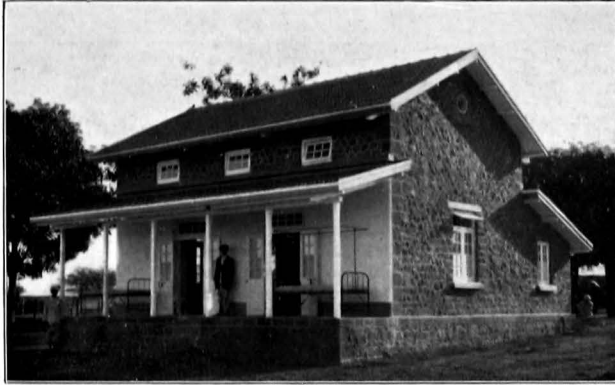
Hospital ward in the new wing at Khondwa, Poona
