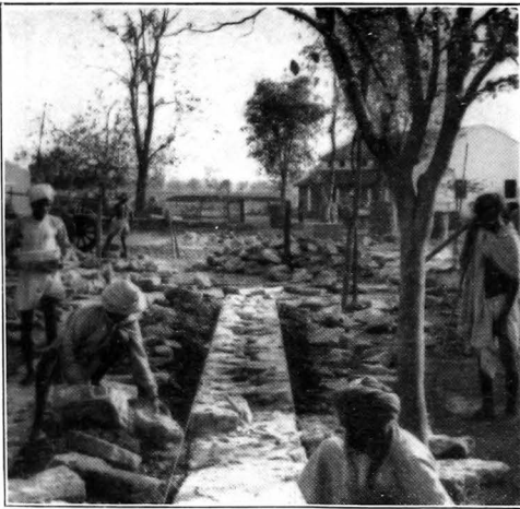
Patients lay foundations for hospital extensions (Chandkuri)
