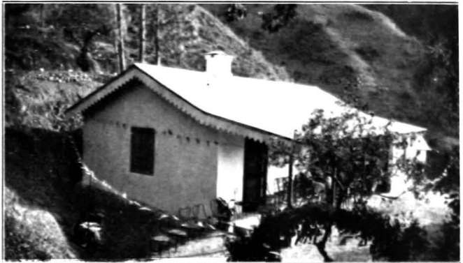
The new Hospital Ward at Subathu
