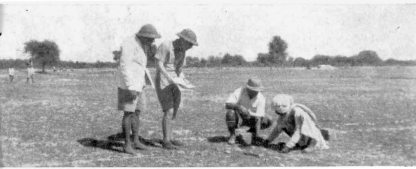
October 1937 Marking out the site
