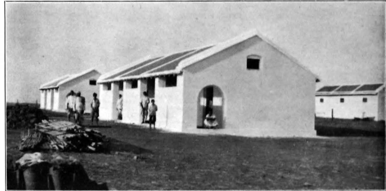
Additional houses recently completed at Shantipur, Dhamtari
