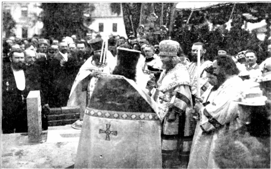
SERVICE AT THE LAYING OF THE FOUNDATION STONE OF A LARGE NEW RUSSIAN CHURCH.
