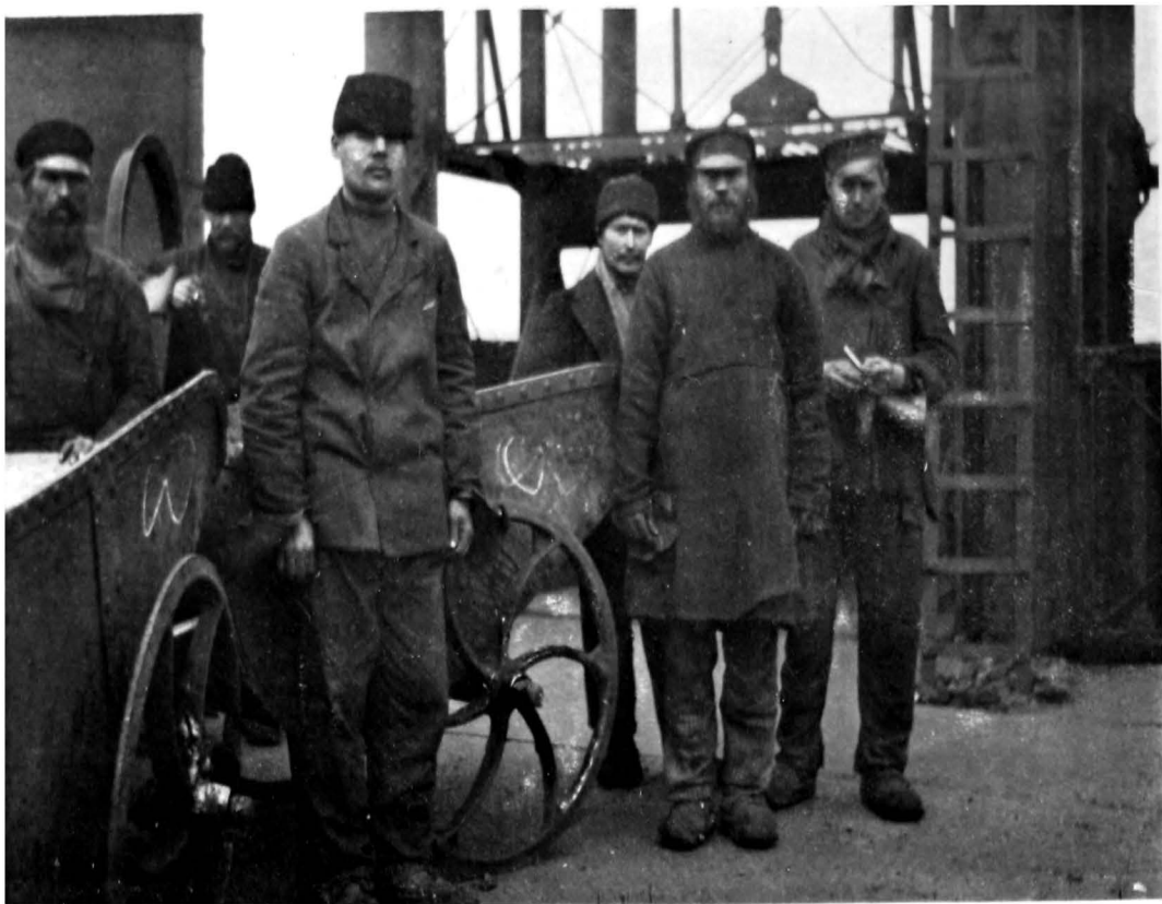
YUZOVO, RUSSIAN IRON-WORKERS ON A BLAST FURNACE.
