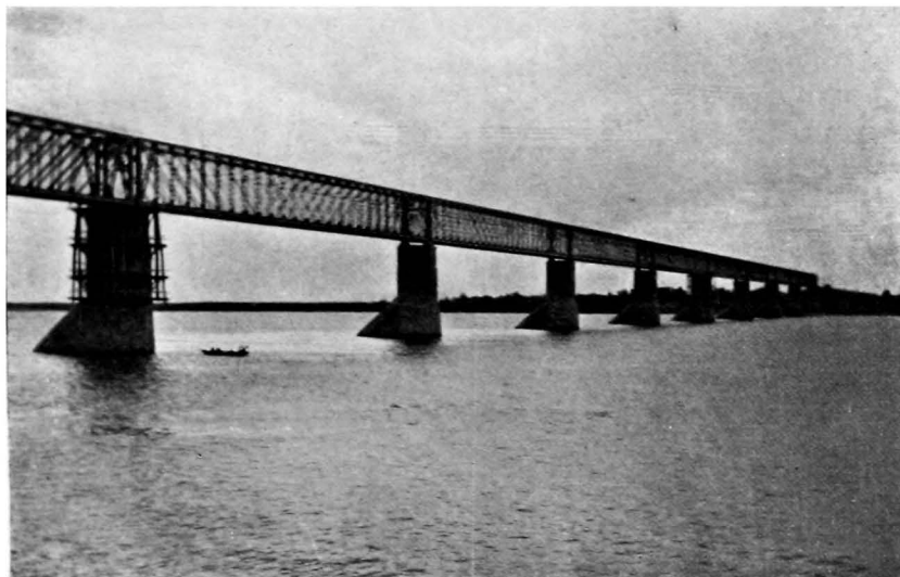
THE ALEXANDER II. VIADUCT AT BATRAKI ON THE VOLGA. THE ONLY BRIDGE ACROSS THE GREAT RIVER BELOW RYBINSK.
