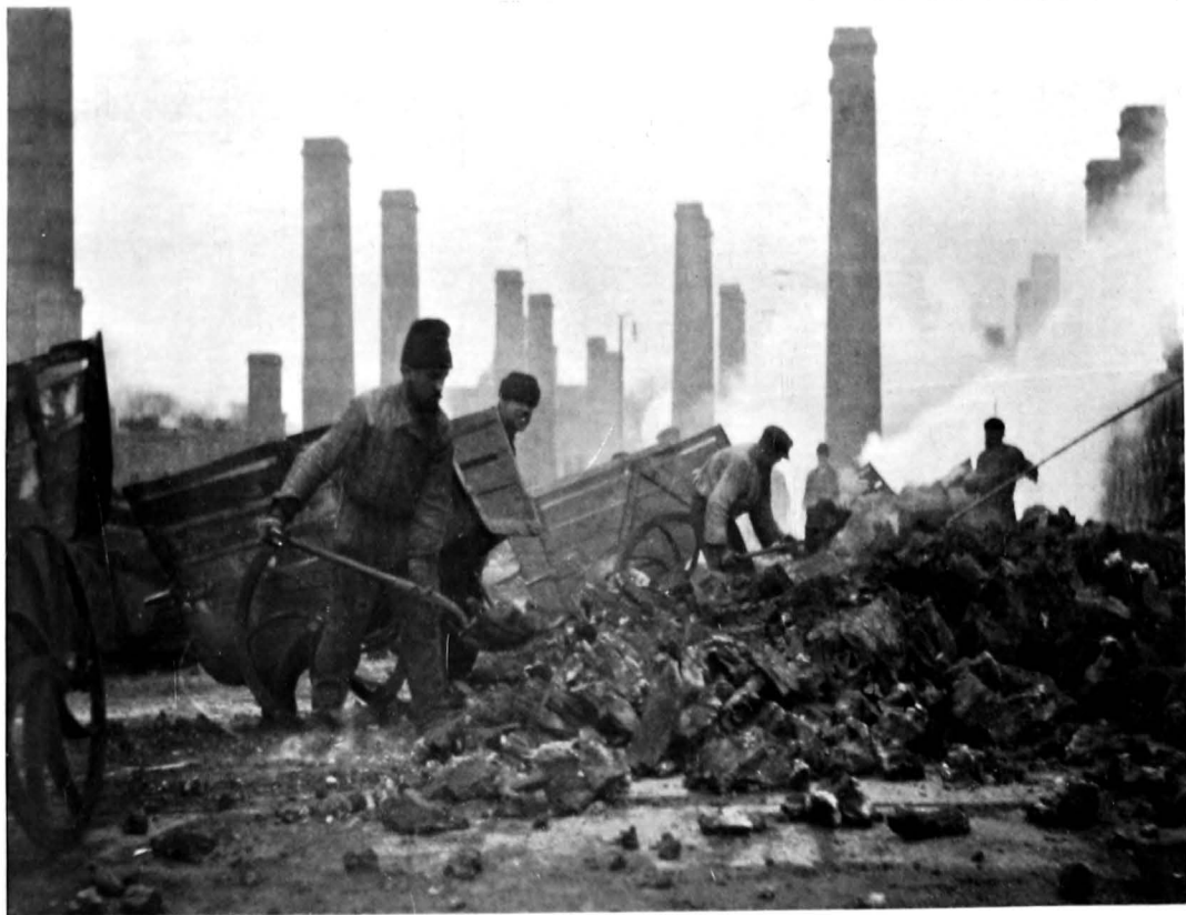
IRON AND STEEL WORKERS.
