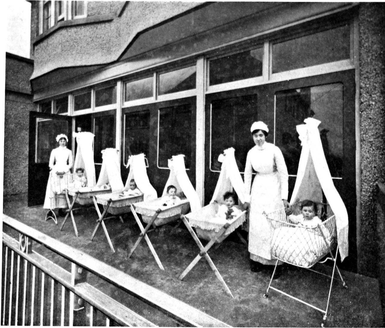
VIEW OF THE BALCONY AT THE LEASOWE BABIES' HOSPITAL.
